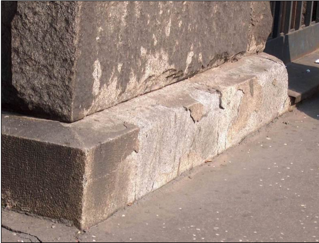
Belgrade, the Post building, southern facade: damages on the granite caused by salt
