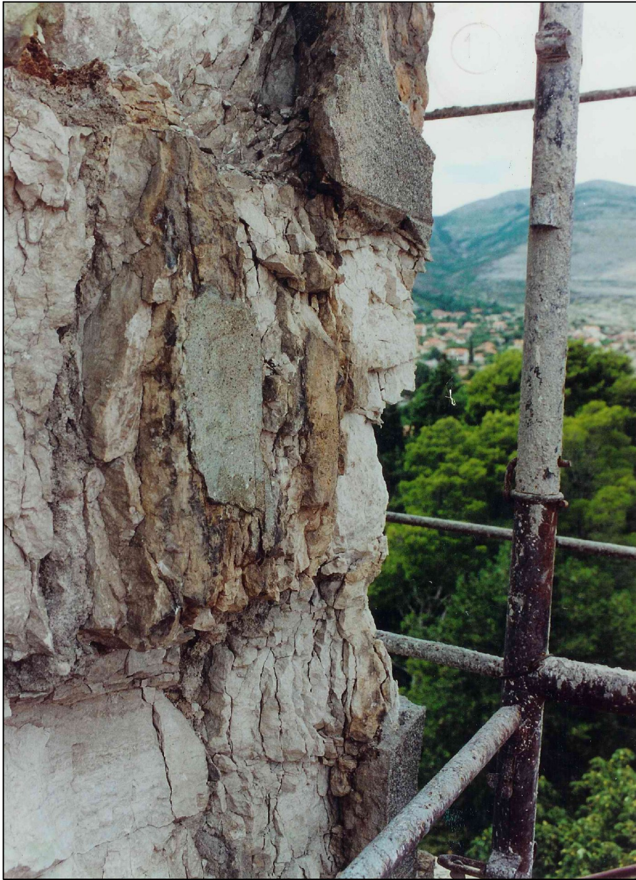
Trebinje, Transfiguration Temple: damage on the limestone
