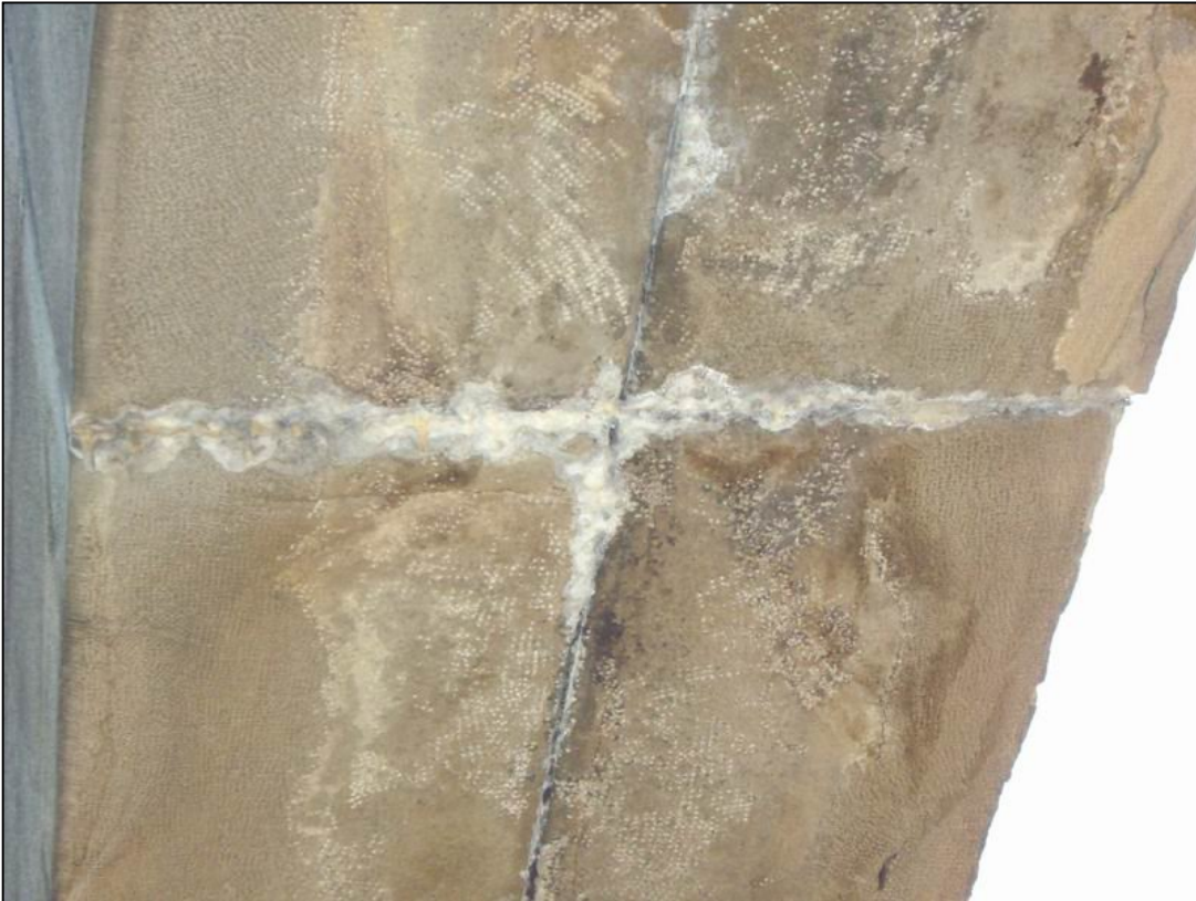
Belgrade, Monument of Belgrade liberators 1944, salting out of sandstone
