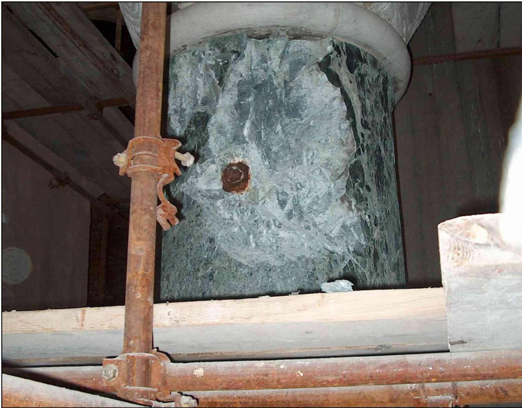
Belgrade, St. Sava Temple: damages on the 'Alpi Verde' marble column caused by corrosion of iron anchor
