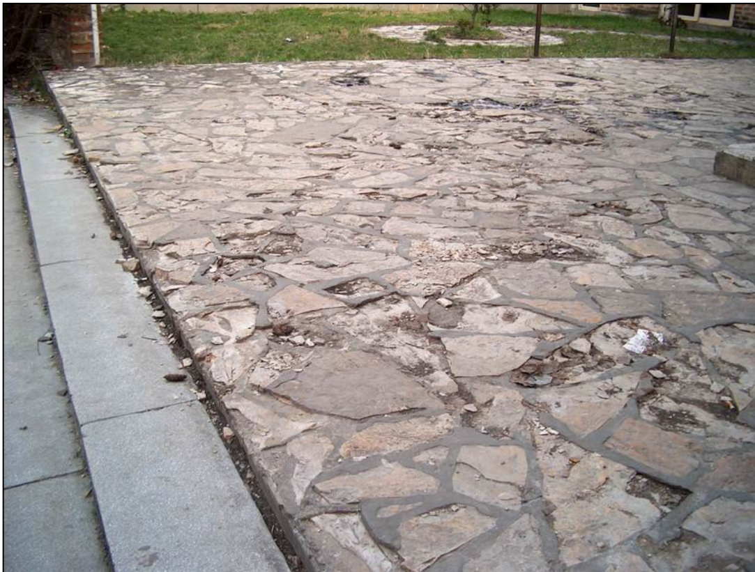
Belgrade, plateau in front of the cinema Sumadija: damages on the 'Struganik' limestone
