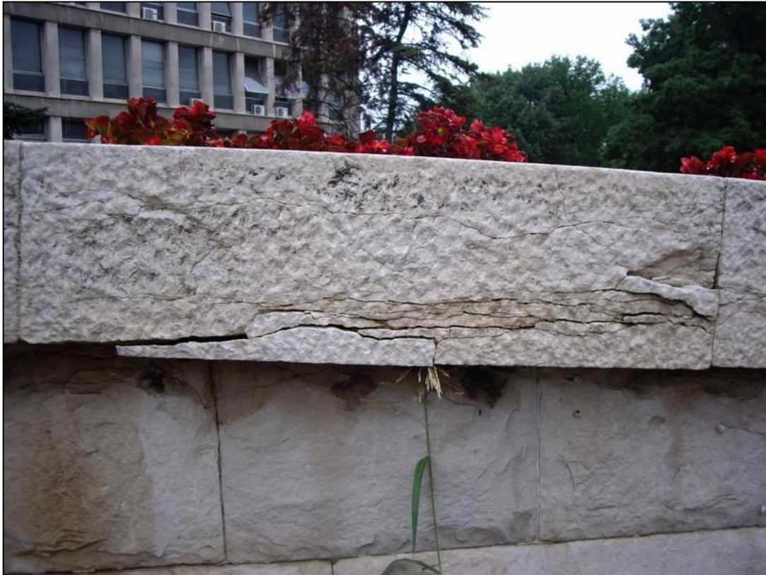
New Belgrade, the building of former Confederal Executive Committee: damages on the 'Brac' marble
