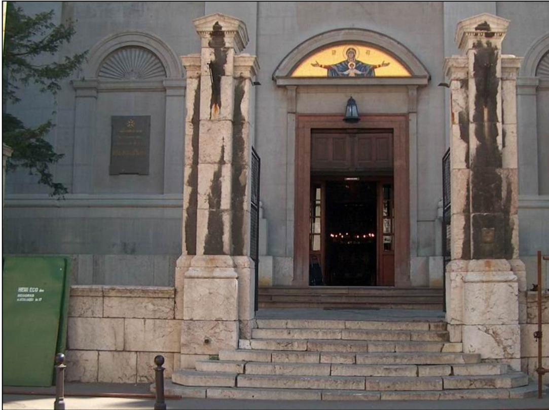
Belgrade, The Temple of Archangel Michael: layers of dirt on pillars of the main gate
