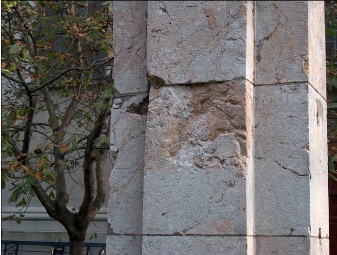
Belgrade, St. Archangel Michael Temple: damage on the breccia caused by rinsing of the binder (clay)
